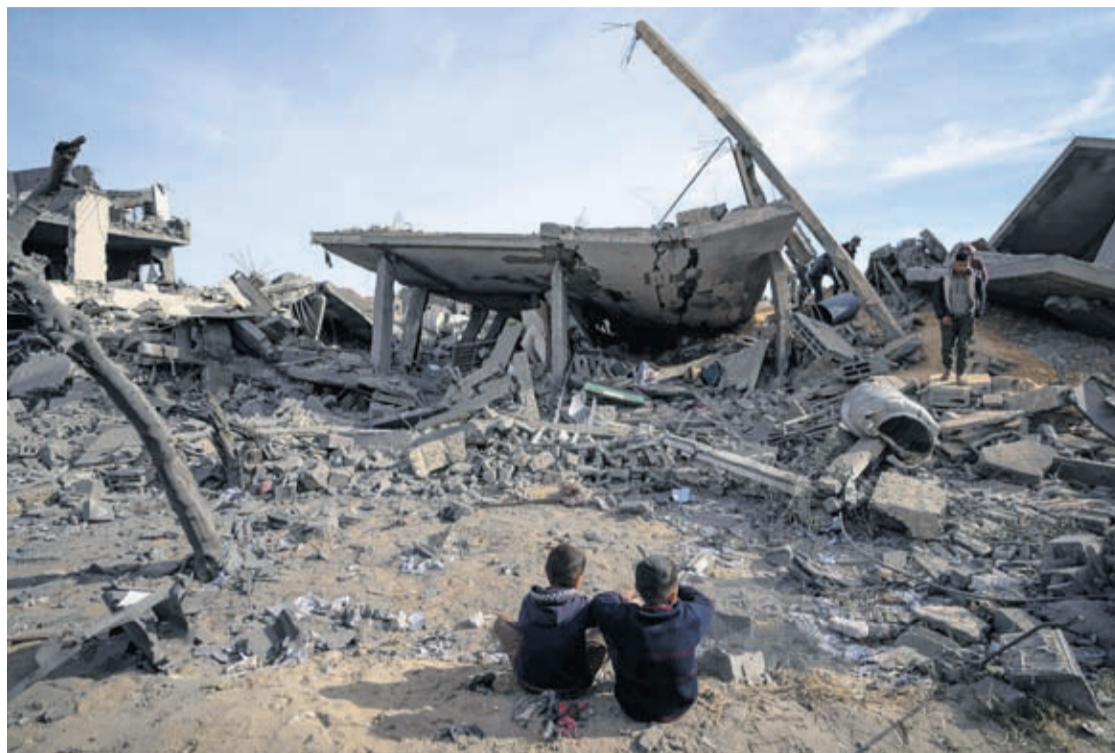
Palestinians inspect the damage to residential buildings where two Israeli hostages were reportedly held before being rescued during an operation by Israeli security forces in Rafah, southern Gaza Strip, Monday, Feb. 12, 2024.
